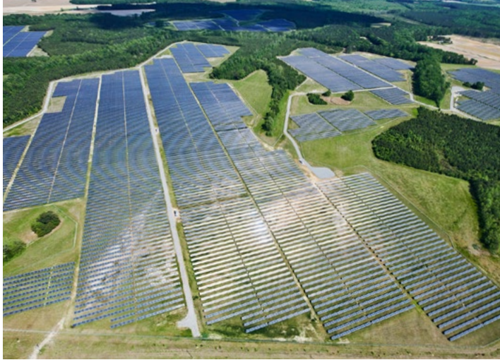
Dominion Energy’s Southampton Solar Farm, consisting of more than 385,000 solar modules on approximately 1,200 acres in Virginia, provides energy to Amazon Web Services.
