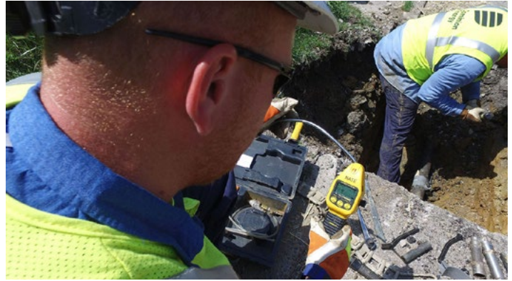
A gas distribution crew performs pipeline testing.
