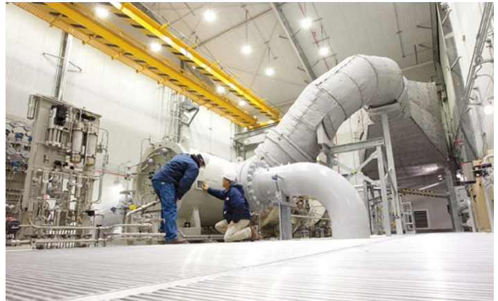
Crews check equipment regularly at gas compressor stations to ensure safe and efficient operations.
