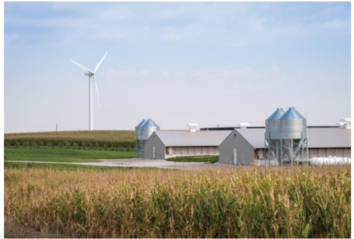
RNG facility in Milford, Utah.
