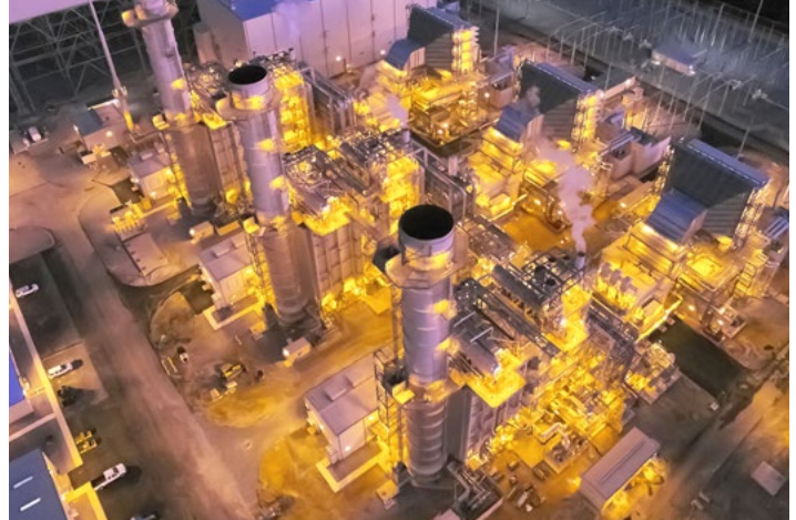
Brunswick County Power Station.
