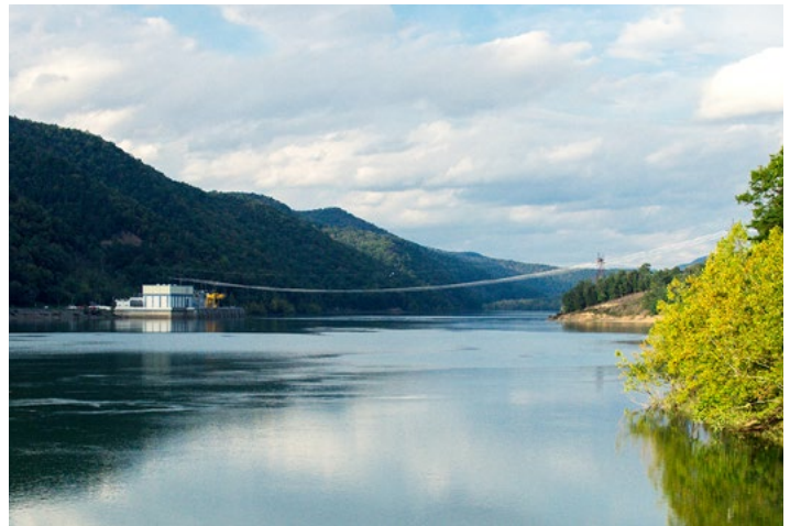
Bath County hydro pumped-storage facility.
