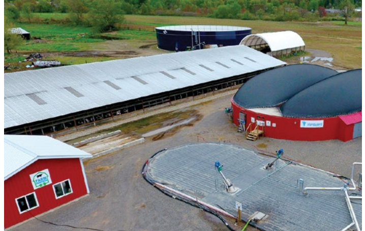
Methane emissions are captured from farming operations for processing into natural gas (photo courtesy of Vanguard).
