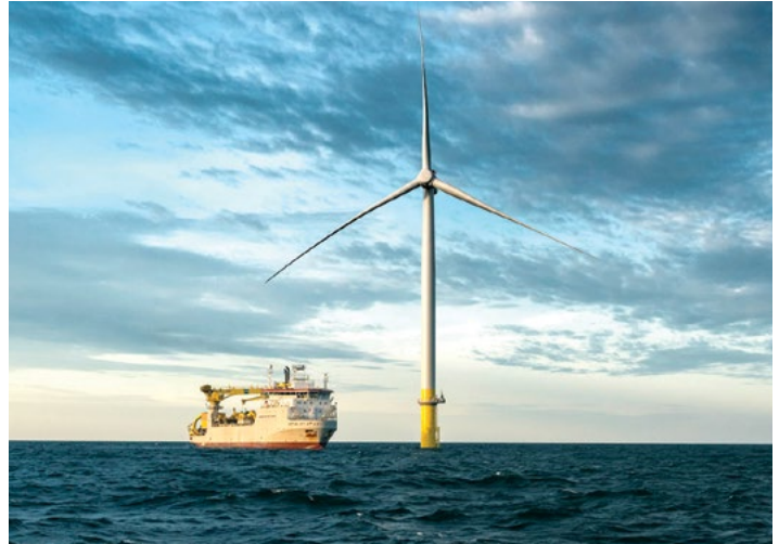
One of the first turbines to be completed for the Coastal Virginia Offshore Wind project.
