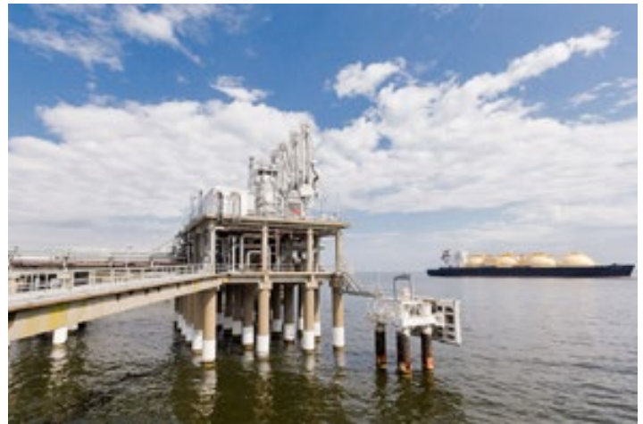
Cove Point LNG Facility.
