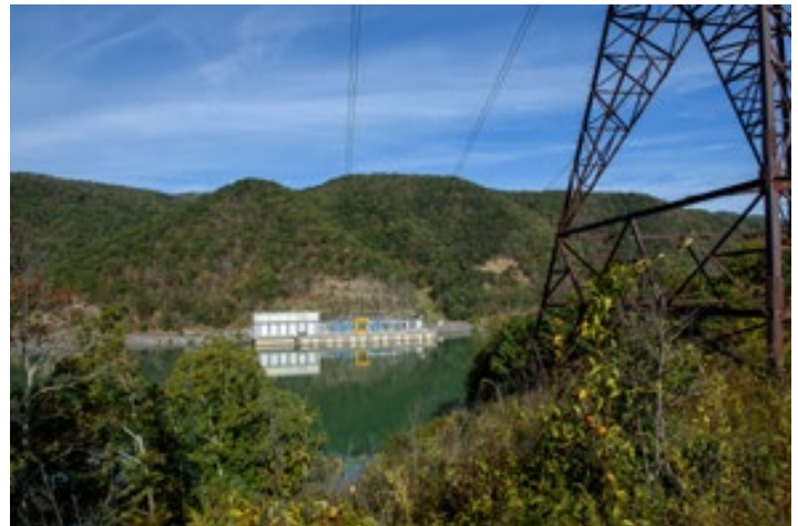
Bath County Pumped Storage Facility
