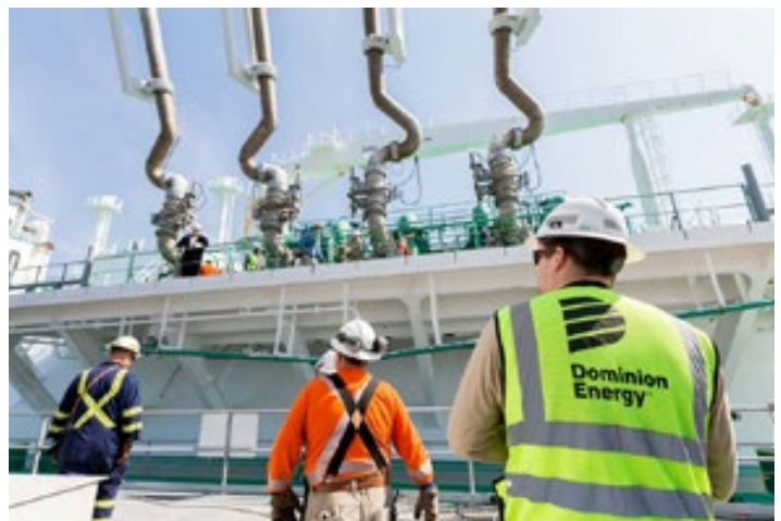
Cove Point LNG Facility.
