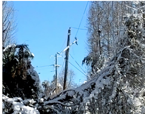
While the crossarms on this line were damaged due to a fallen tree, the pole itself remained intact – a function of our “main feeder” hardening program.
